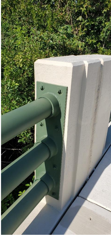
Typical pipe rail support bracket assembly.
