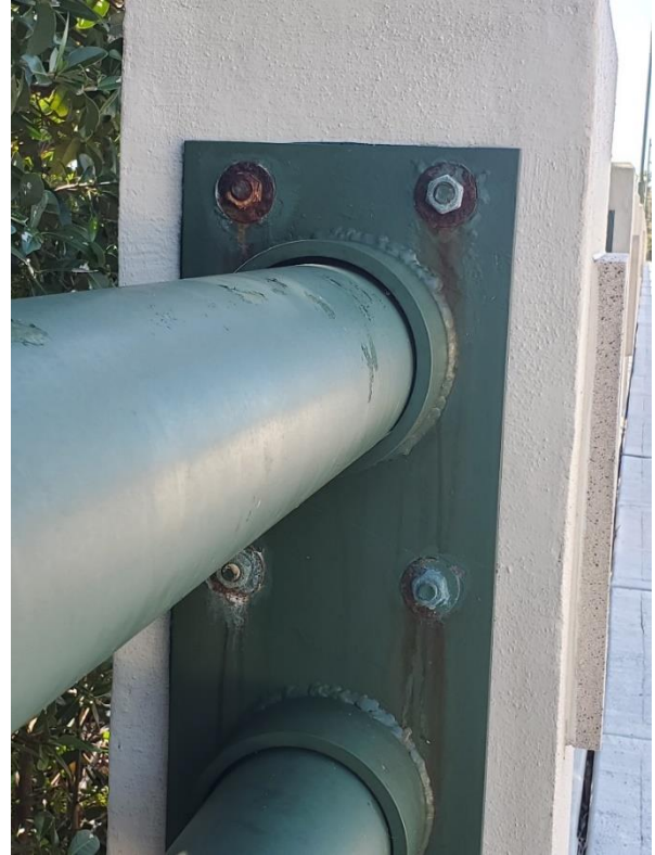
Several pipe railing support bracket assemblies showing limited deterioration at bolting.
