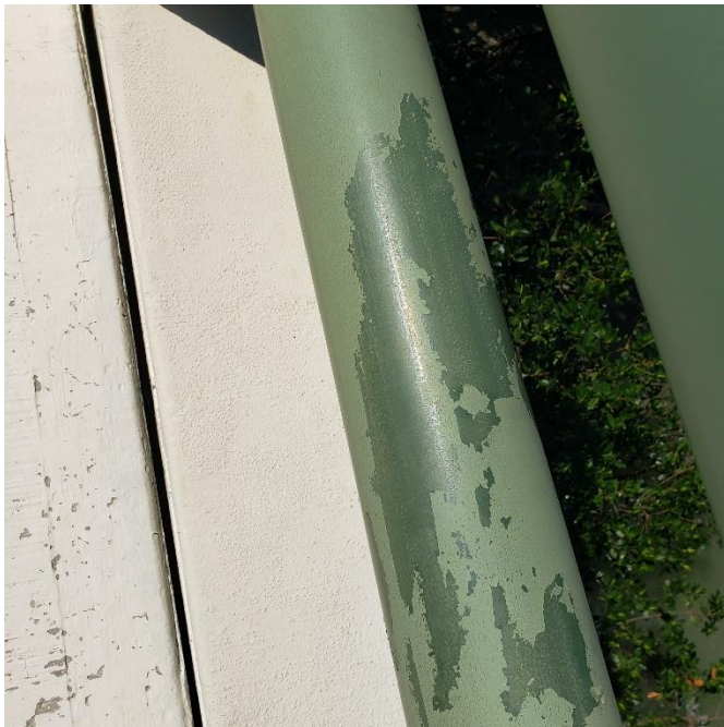
Typical pipe rail fading and peeling paint. Note previous coating underneath.
