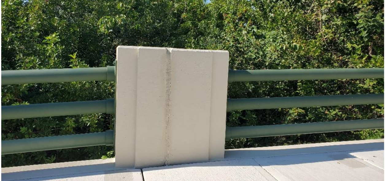
Double pipe support at pile bent location. Area between individual support provides for movement.
