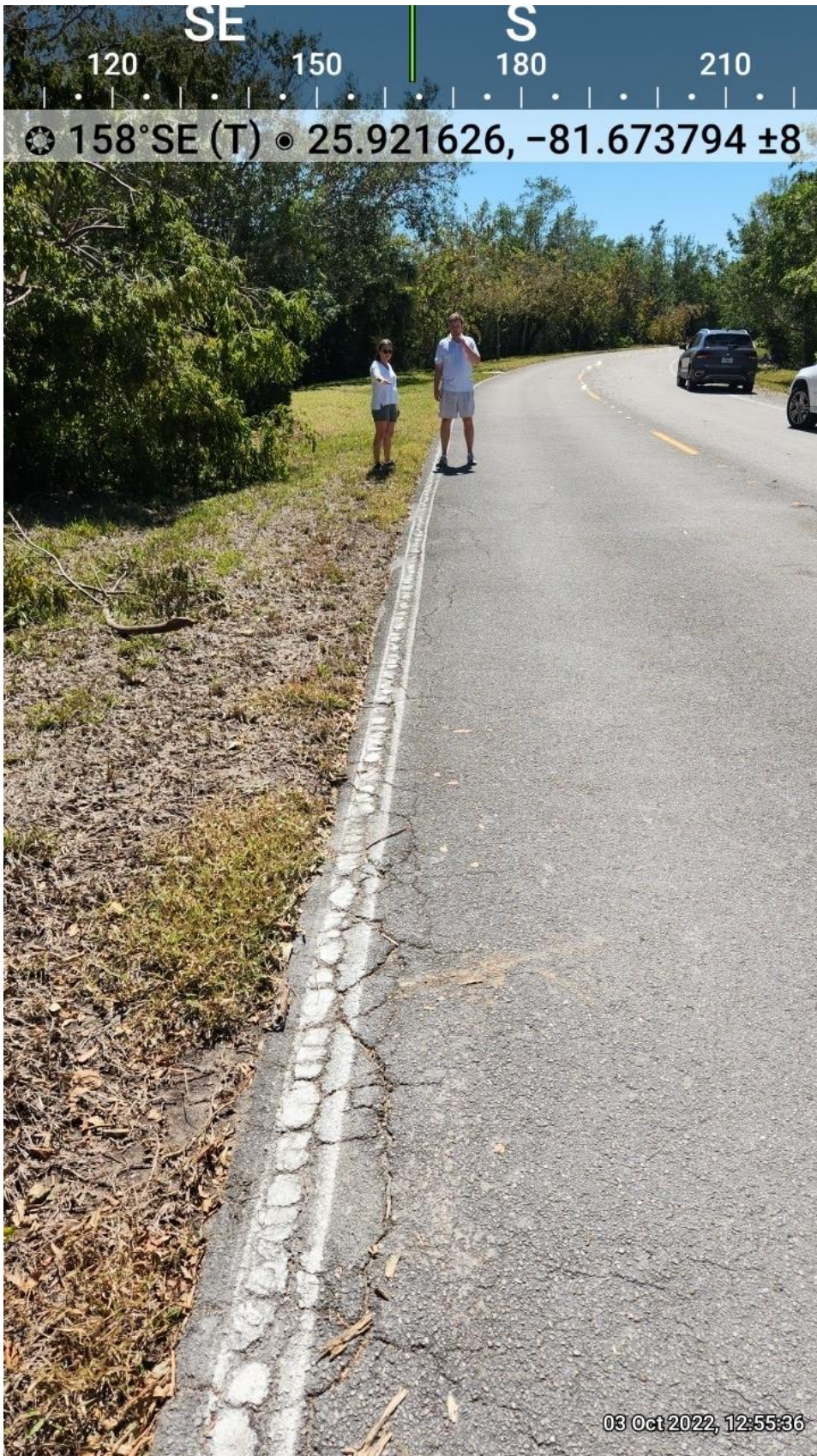
Excessive alligator cracking in road.
