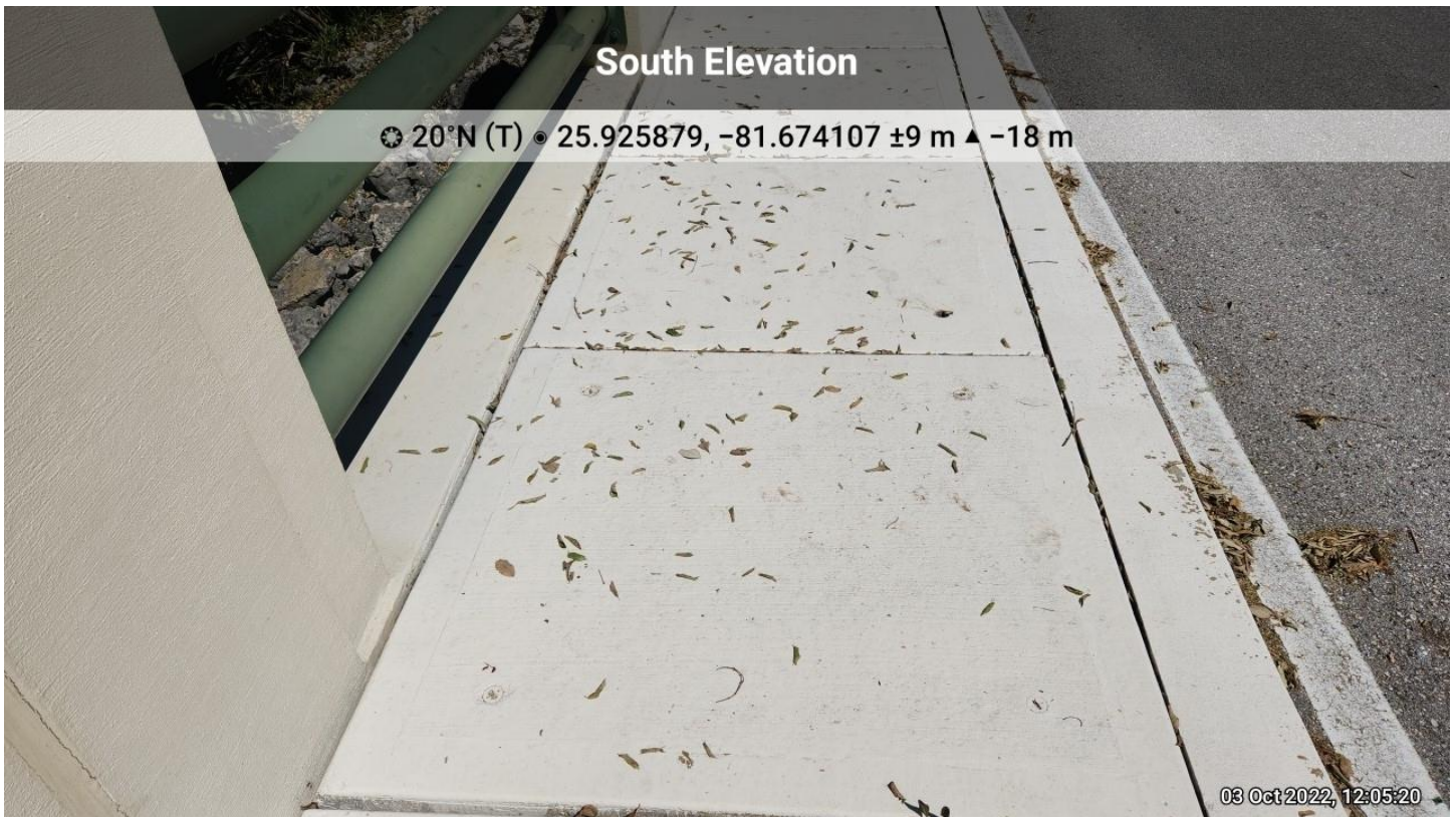
Loose sidewalk panel.
