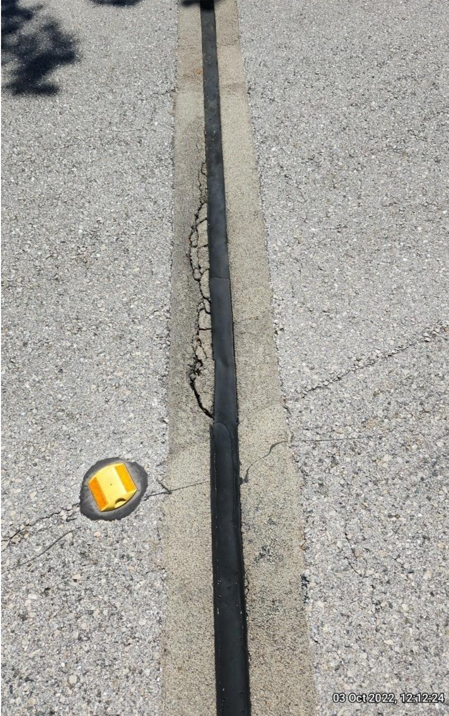
Cracking in bridge joints, span 11.
