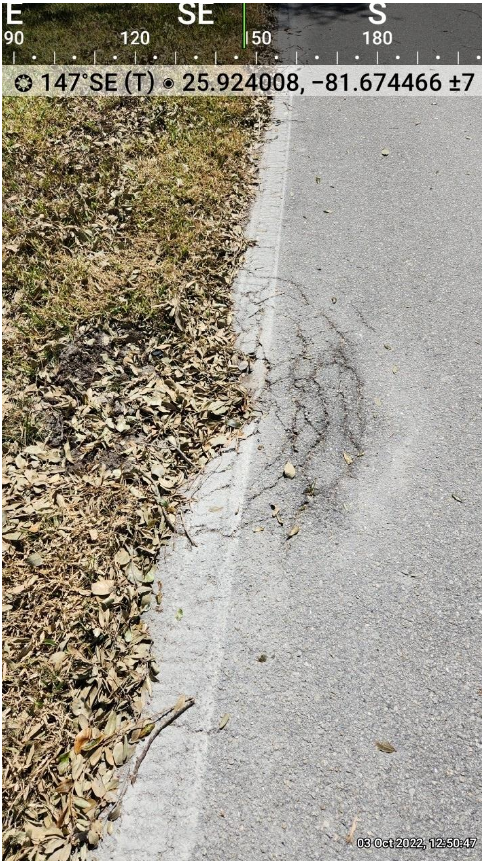
Broken irrigation head and cracking in road. 300' southeast from bridge.
