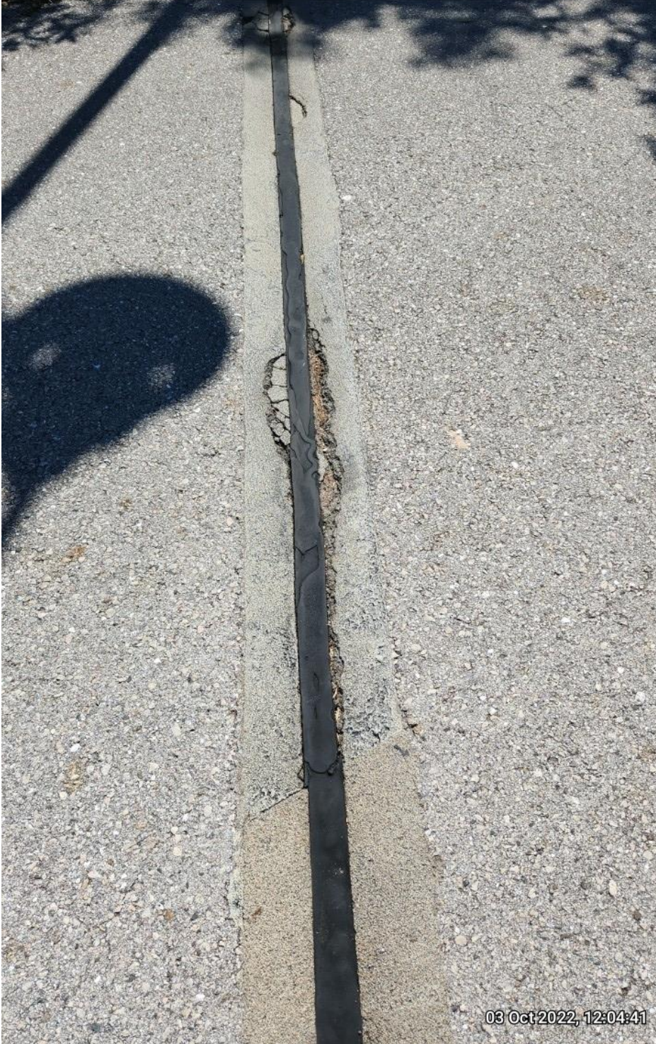
Cracking in bridge joints, span 1.
